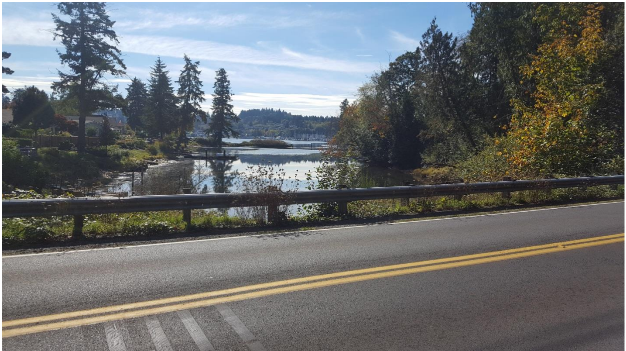
Photo #10: Looking south at Gig Harbor bay over Vernhardson Street. Crescent Creek discharges to bay through culvert underneath road.
