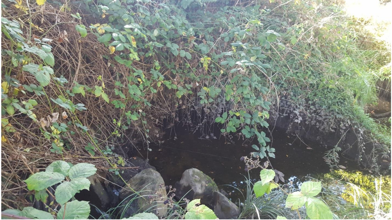
Photo #9: Looking south towards culvert underneath Vernhardson Street at south end of pond.
