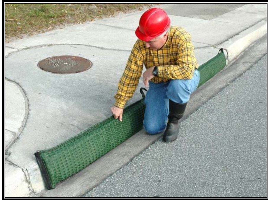
Figure 4.20. Commercially Available Gutter Guard Being Replaced.
