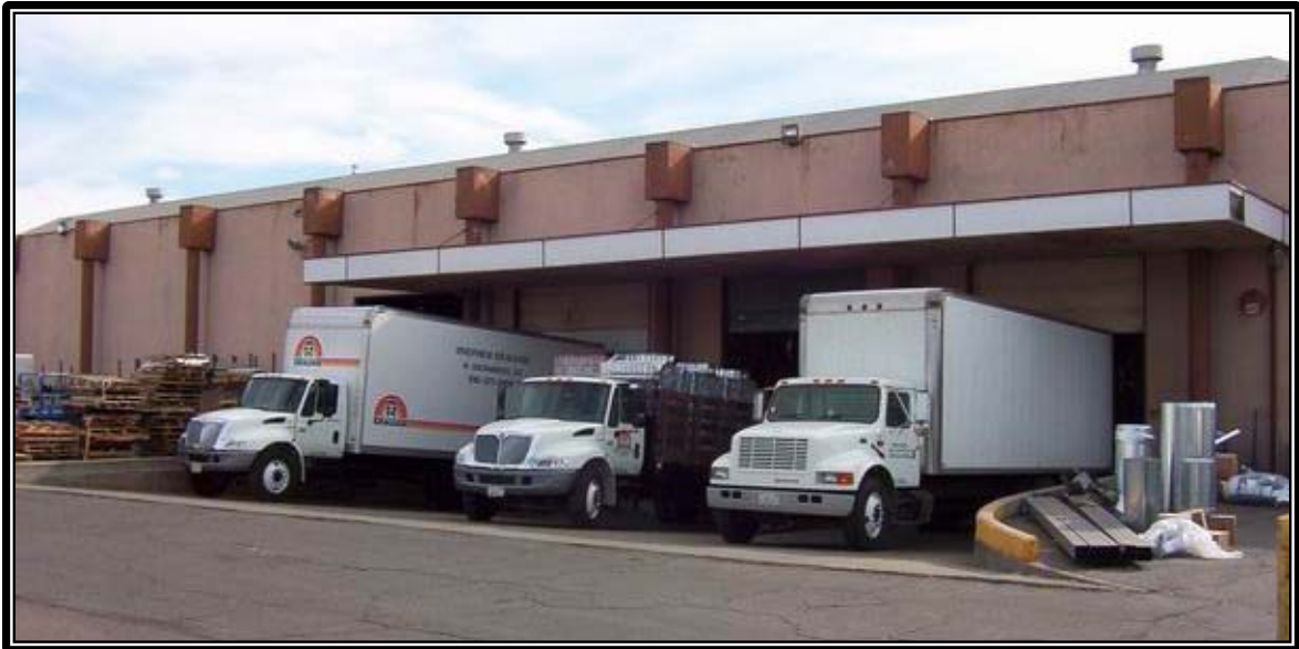
Figure 5.2. Loading Docks with an Overhang to Prevent Material Contact with Rainwater.
