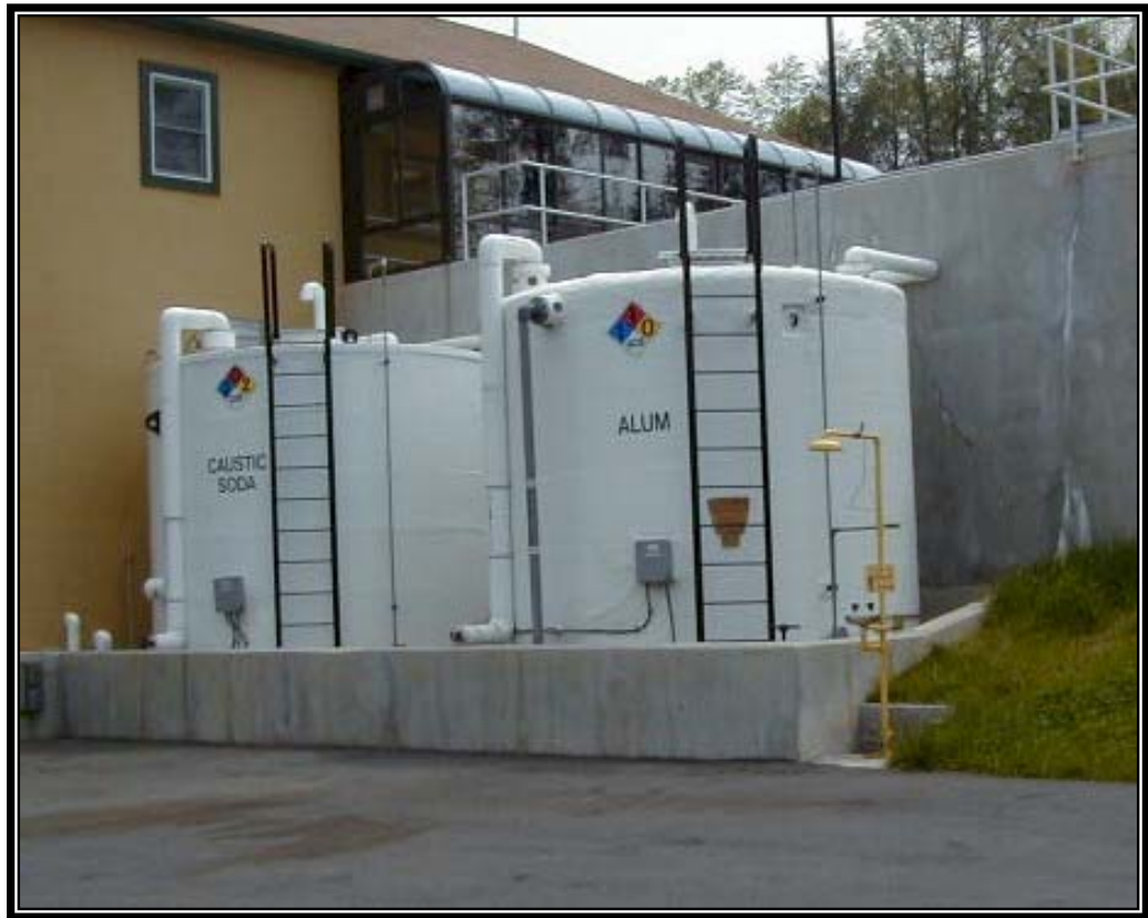
Figure 4.19. Aboveground Storage Tanks with Secondary Containment.
