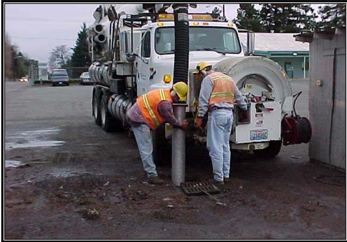
Figure 5.8. Catch Basin Cleaning with a Vacuum Truck.
