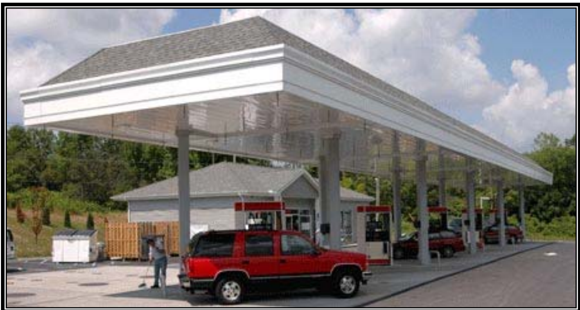
Figure 5.3. Roof at Fueling Island to Prevent Stormwater Runon.
