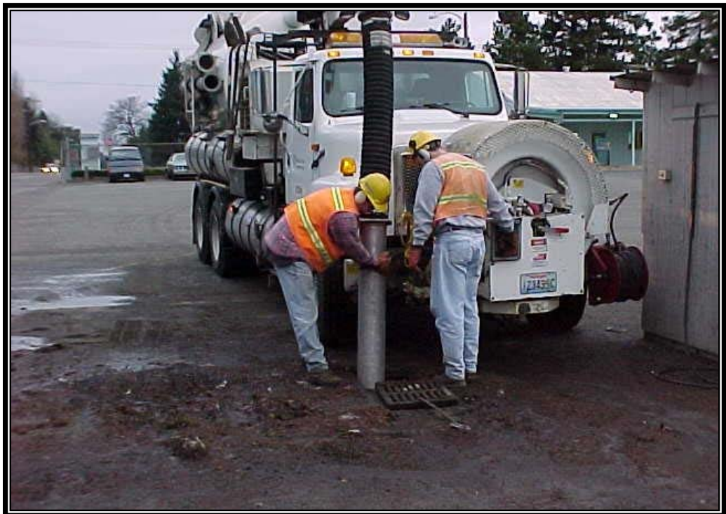
Figure 4.23. Catch Basin Cleaning with a Vacuum Truck.
