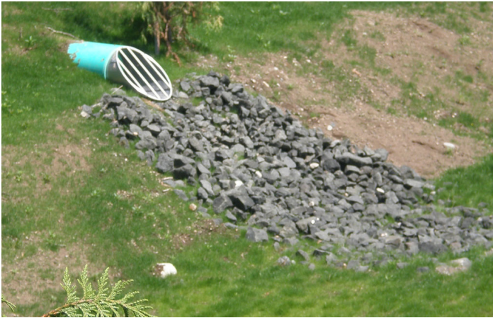
This energy dissipator is in good condition.
