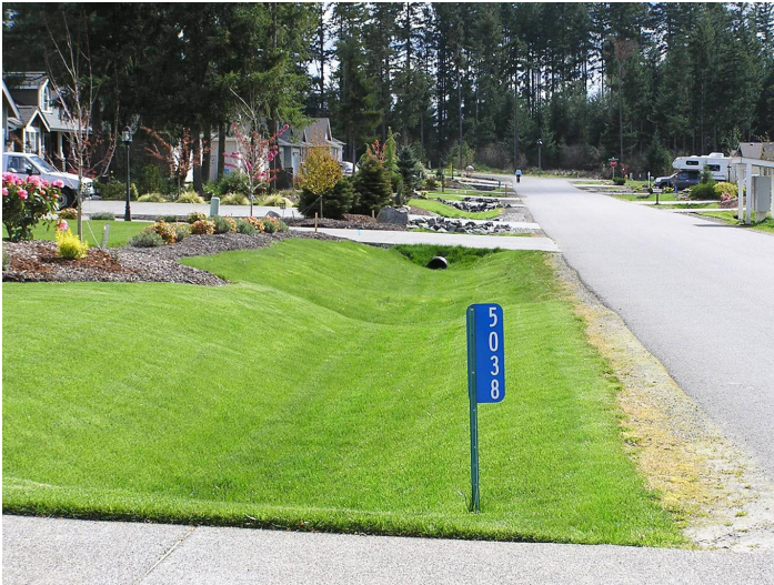
A well-maintained bioswale
