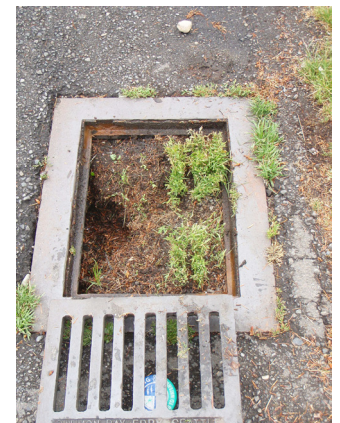
Catch basin clogged with sediment and debris
