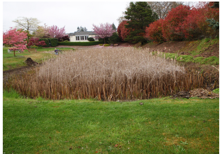
This wet pond is overgrown with cattails. Cattails can cause build-up and reduce pond capacity and should be thinned regularly.
