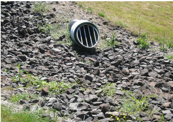
A well-maintained inlet pipe
