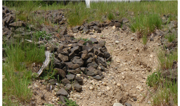
Erosion damages this dissipator.
