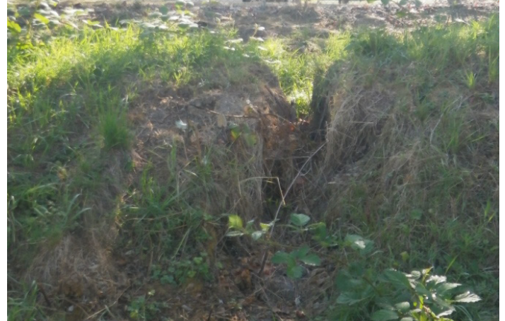
This berm is experiencing erosion.
