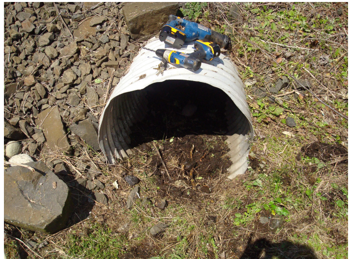
This inlet is loaded with sediment.
